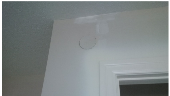
Figure 23: Install the gypsum & finish the wall
