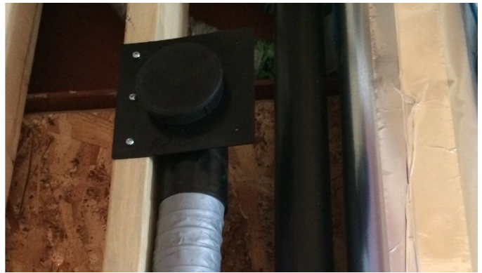
Figure 22: Attach the collar on the wall stud
