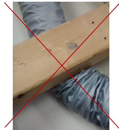
Figure 9: Do not crush the flex duct
