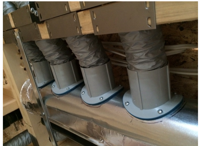
Figure 21: Screw the saddle on the trunk
