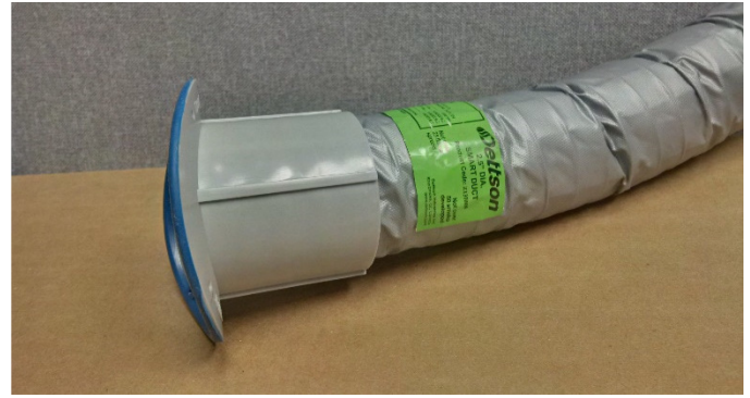
Figure 20: Screw the 2.5" flex into the saddle
