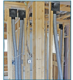
Flex ducts fit inside wall cavity
