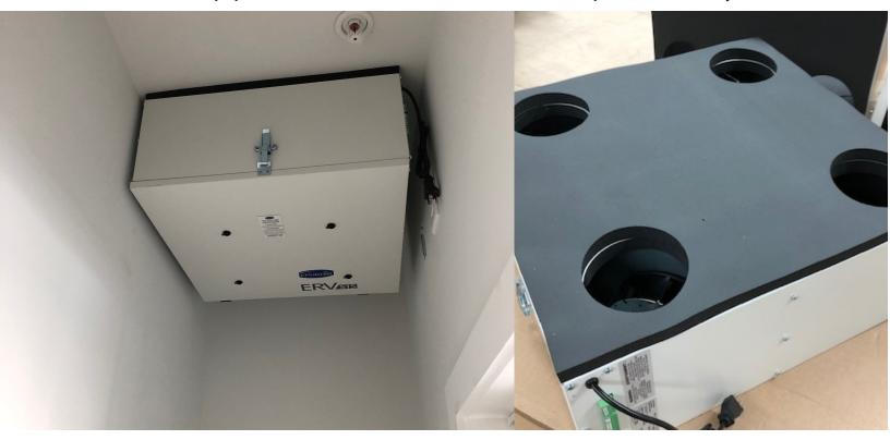
SA-P5R steel mounting plates allow models with foam top ports to be attached directly to the ceiling without the need for flexible ducts.
