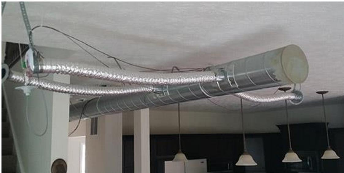
*At its laboratory home in Pittsburgh, IBACOS tested the performance of a heating system that utilized 2.5-inch-diameter ducts for branch runs.*
